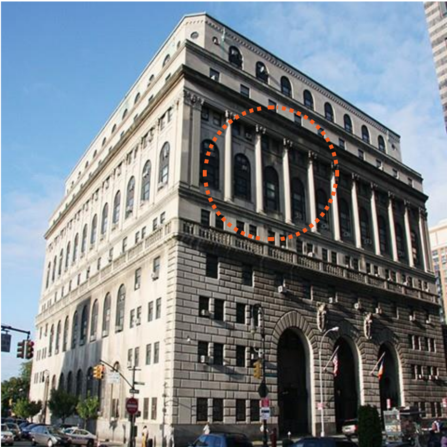
KINGS COUNTY CRIMINAL COURTHOUSE
