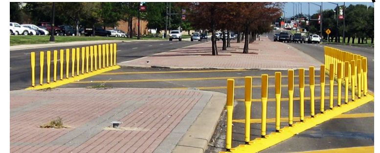
Installation of Traffic Dividers
