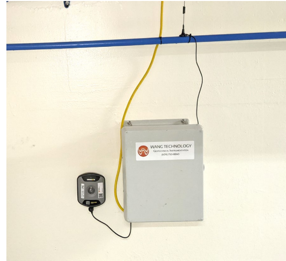
Vibration monitor installed in basement
