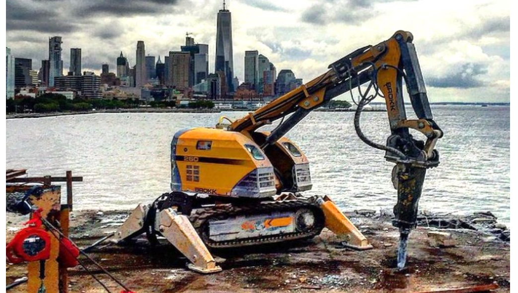
Primary Dismantle Equipment – Electric Brooks
