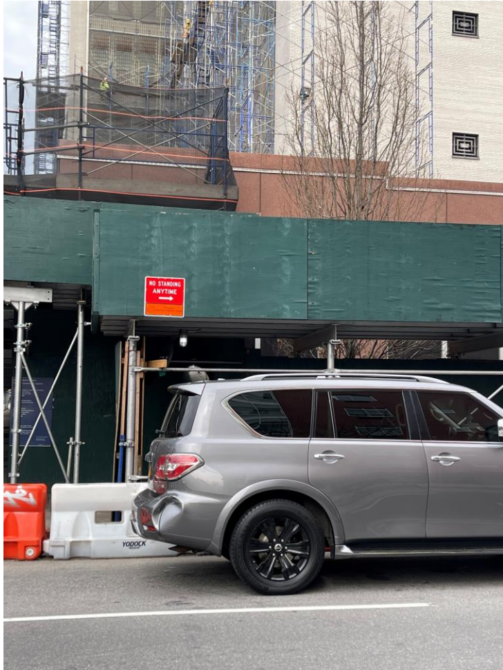
Smith St. No Parking Signs (3/21/23)
