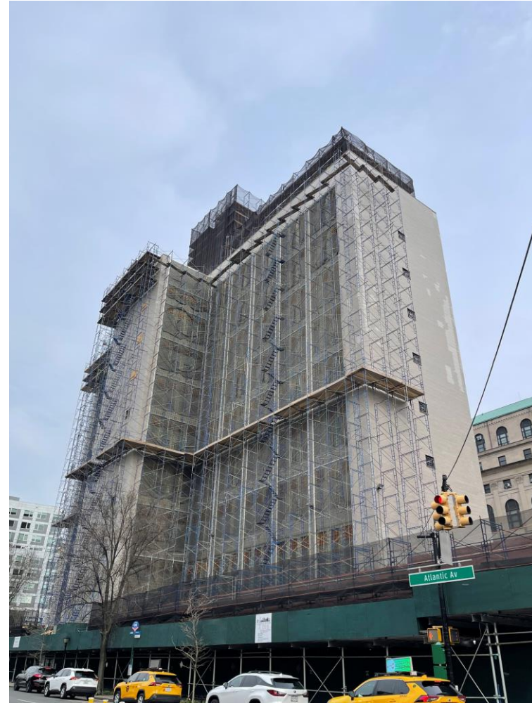
Tower Scaffolding Progression (3/31/23)
