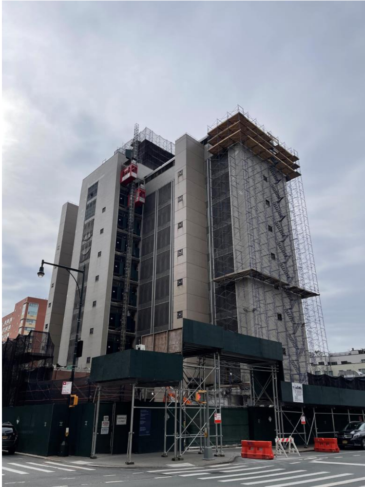
Tower Scaffolding Progression (3/31/23)
