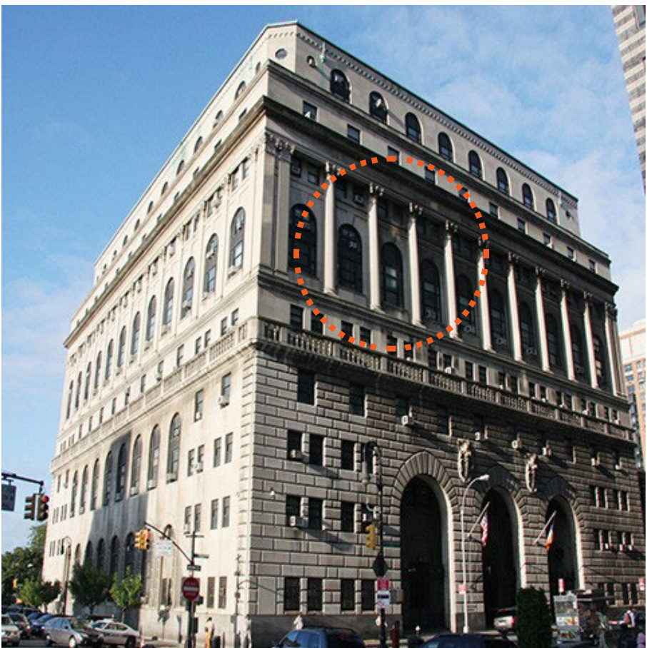
KINGS COUNTY CRIMINAL COURTHOUSE
