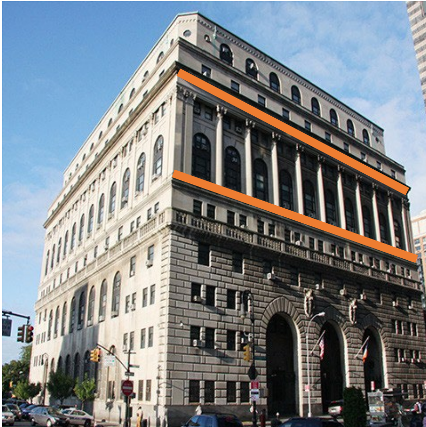
KINGS COUNTY CRIMINAL COURTHOUSE
