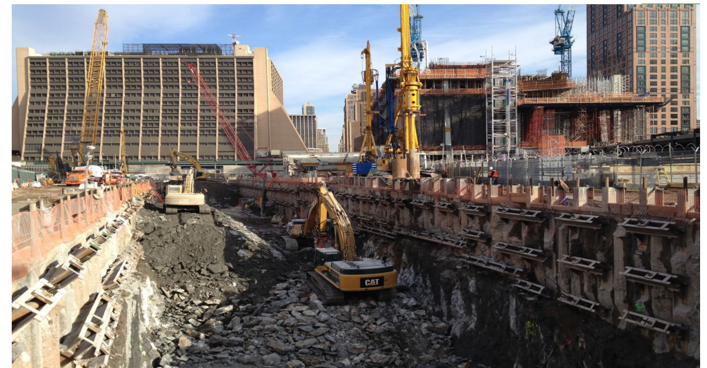
SOE installation adjacent to live train tracks at Hudson Yards
