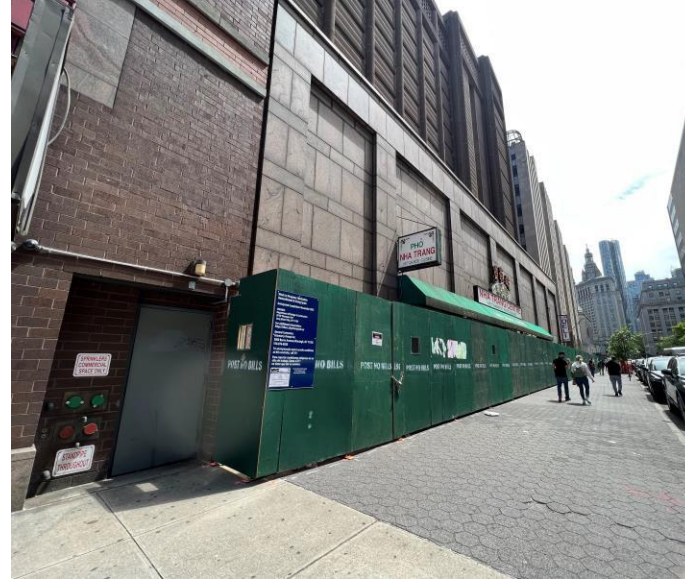
Site Protection Fence on Centre Street (7/21/2022) Centre Street/中央街保護圍欄(7/21/2022)
