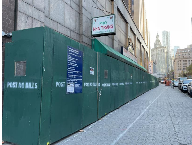
Site Protection Fence on Centre Street (11/21/2022) Centre Street/中央街保護圍欄 (11/21/2022)
