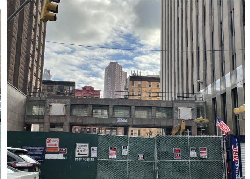
White Street Bridge Dismantle (12/12/2022) 拆除白街行人天橋 (12/12/2022)
