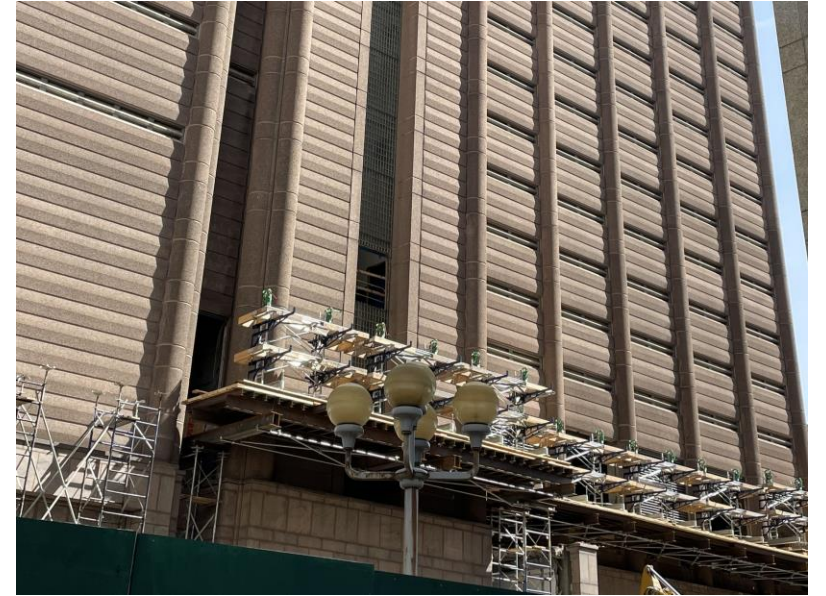
North Tower Scaffolding Installation (4/11/2023)
