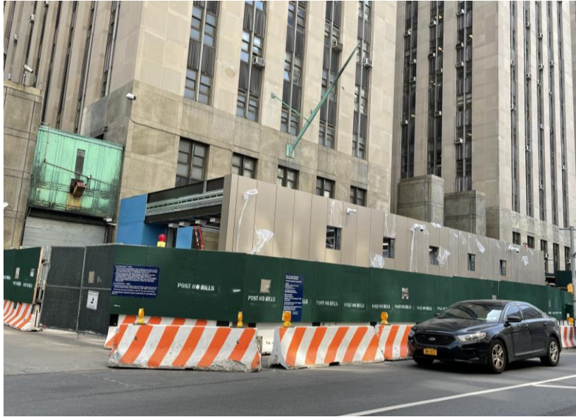
Interim Sally Port Construction (4/11/2023)
