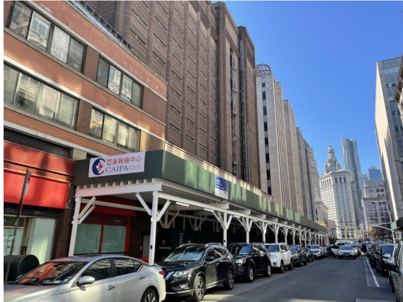
Sidewalk Shed Installation on Centre Street (4/3/2023)
