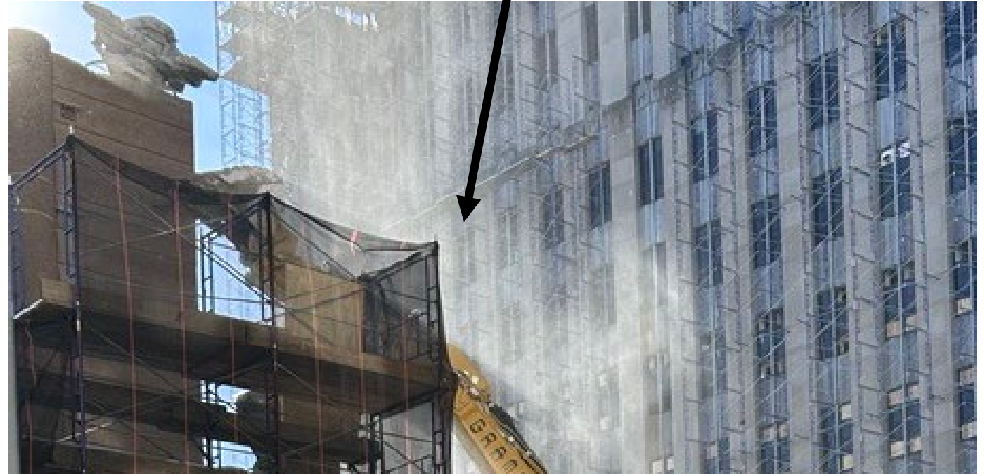
Mist used for dust mitigation
