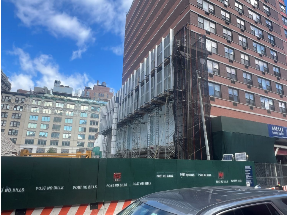
North Tower Gym Wall Scaffolding (6/24/2024)
