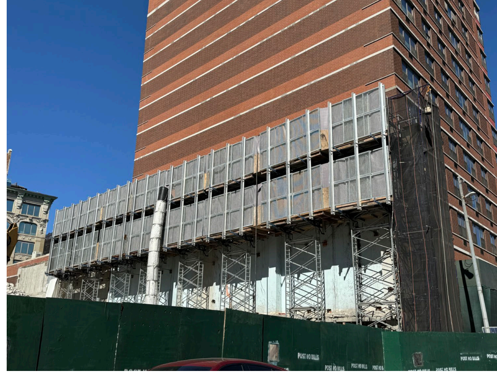
North Tower Gym Wall Scaffolding (10/10/2024)
