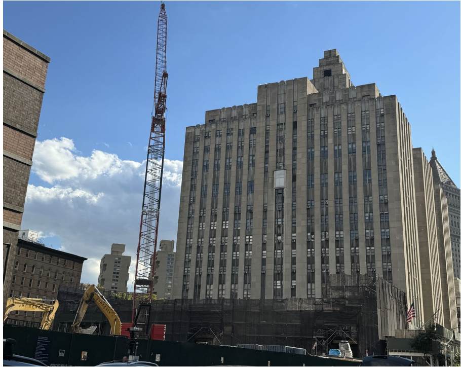
South Tower Dismantlement Progress (10/9/2024)
