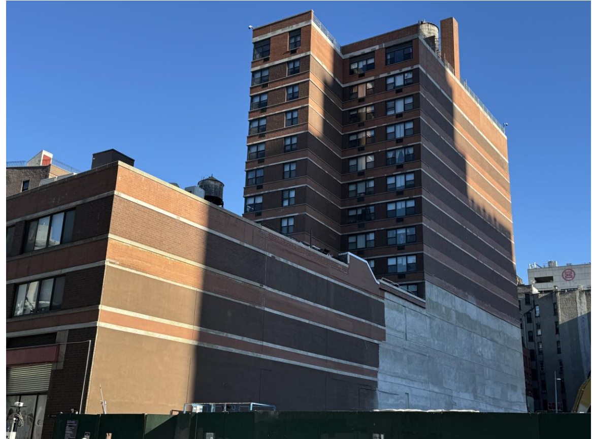
North Tower Gym Wall Scaffolding (12/13/2024)
