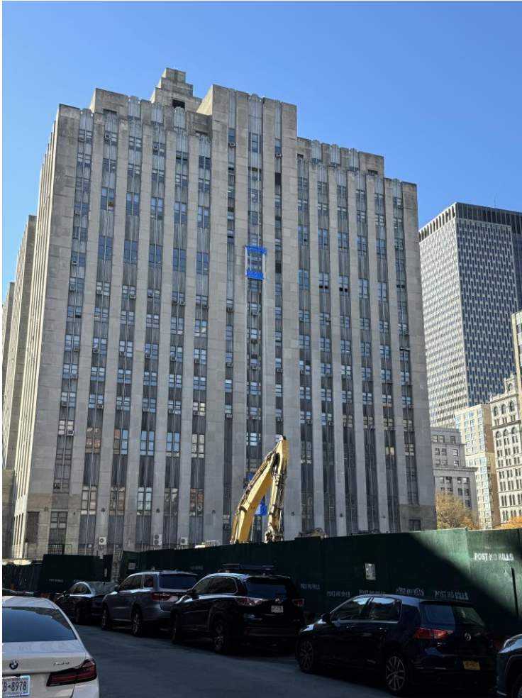
South Tower Dismantlement Progress (12/13/2024)
