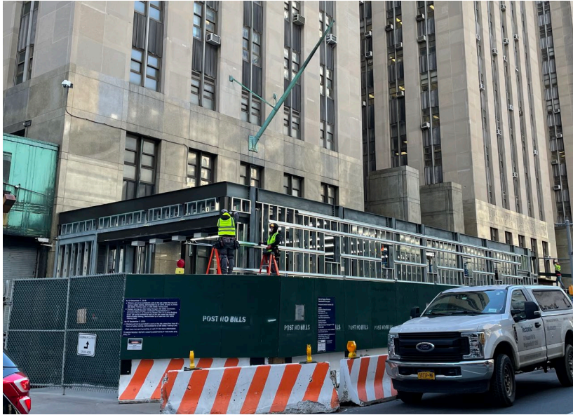
Interim Sally Port Construction (2/14/2023)
