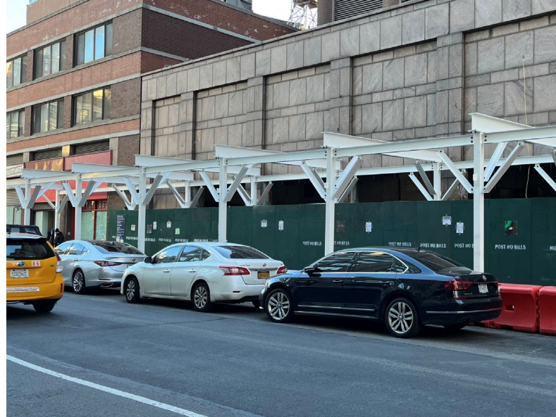
Sidewalk Shed Installation on Centre Street (2/14/2023)
