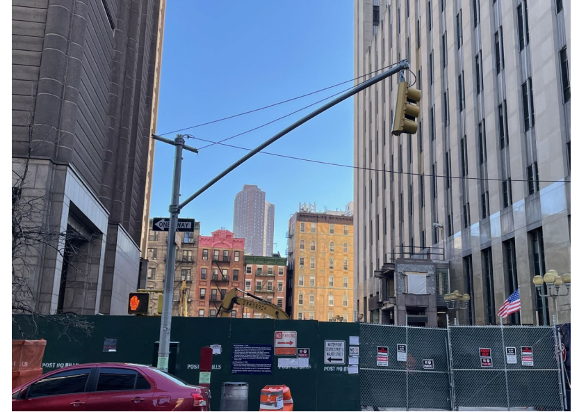
White Street Bridge Dismantle Completed (2/14/2022)
