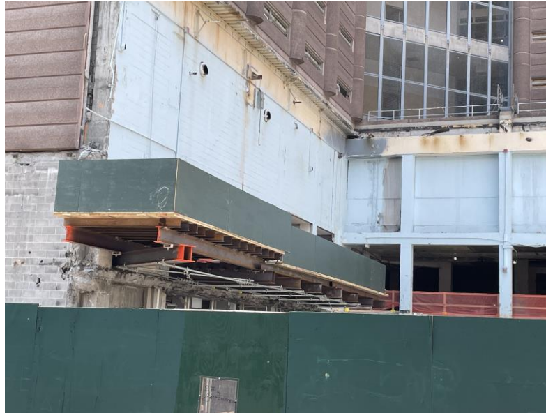
Needle Beams Installation on Baxter Street (6/19/2023)
