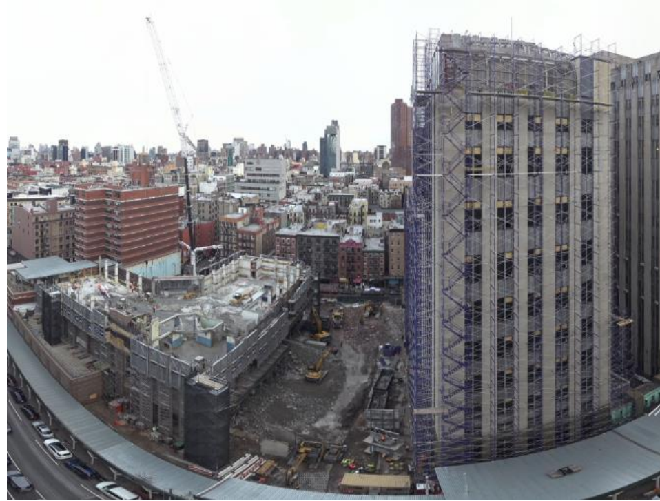
North Tower and South Tower Scaffolding Installation (01/12/2024)
