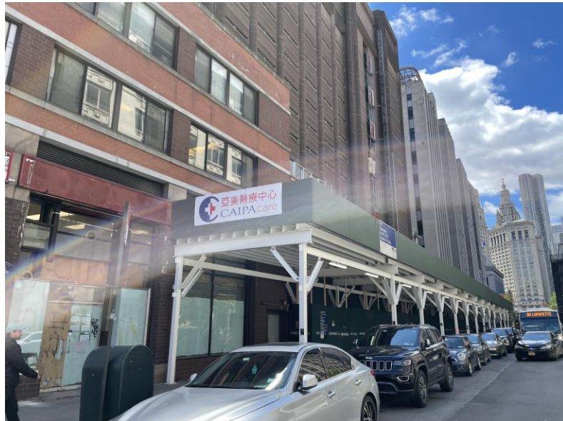
Sidewalk Shed Installation on Centre Street 中央街人行道棚(5/5/2023)
