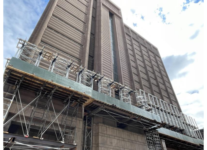
North Tower Scaffolding Installation 北樓安裝鷹架 (5/5/2023)
