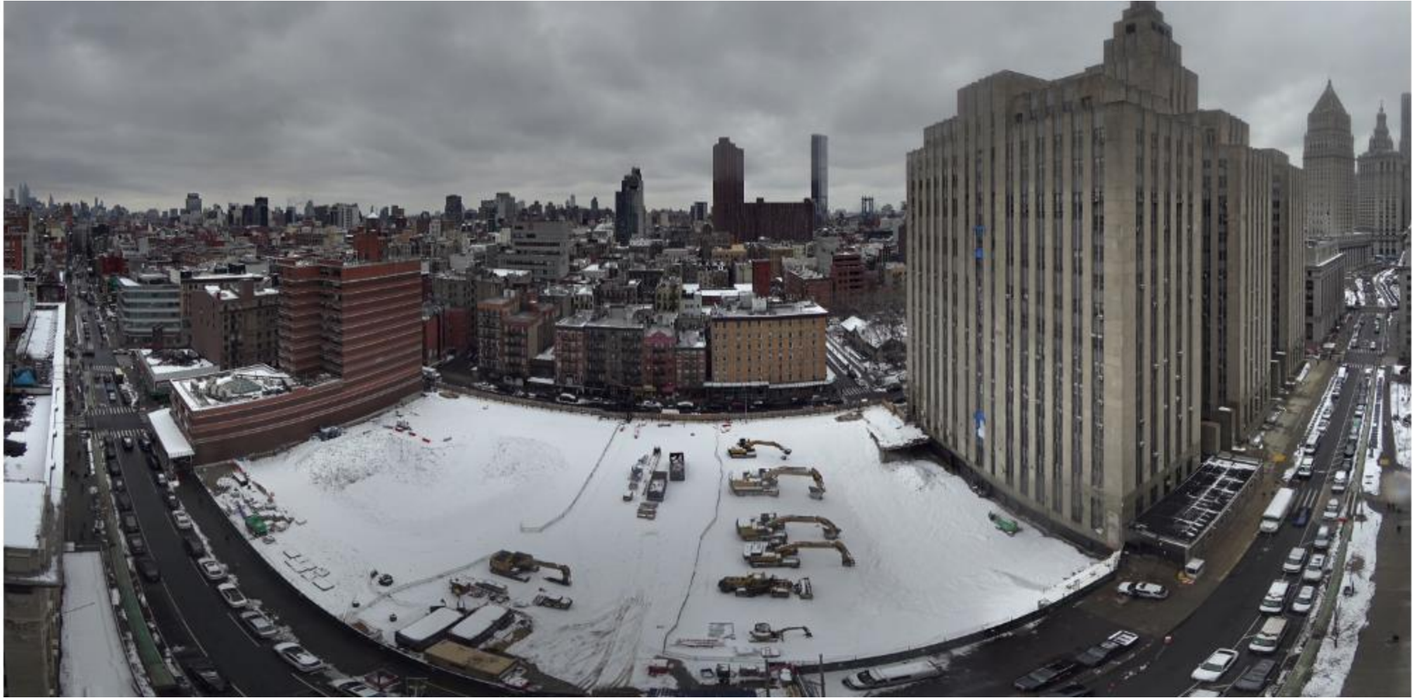
Site Preparation and Chung Pak Wall Waterproofing (2/12/2025)
