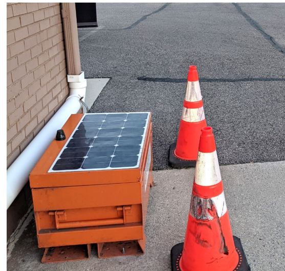
Vibration monitoring installed outside on sidewalk
