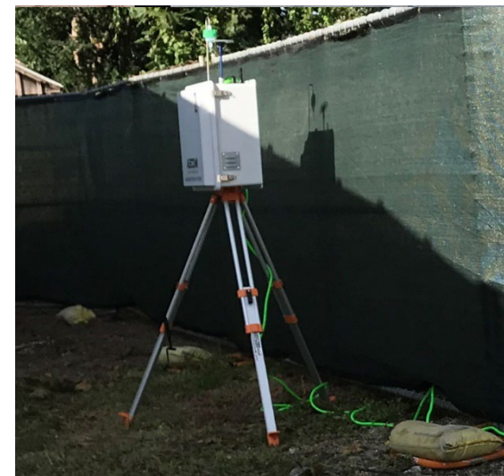
Air Quality monitor installed close to site fence 安裝在工地圍欄附近的空氣質量監測儀
