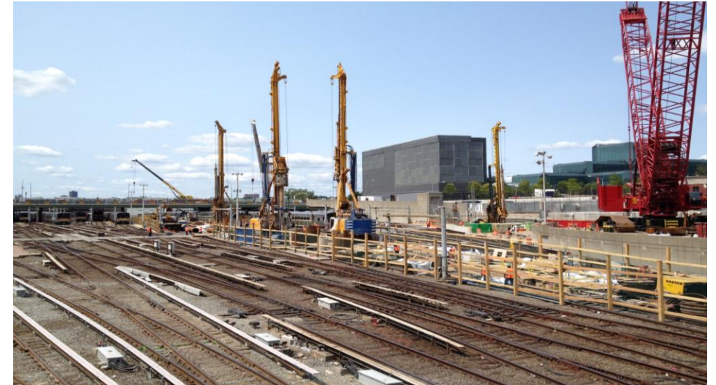
Pile Driving successfully adjacent to live train tracks at Hudson Yards
