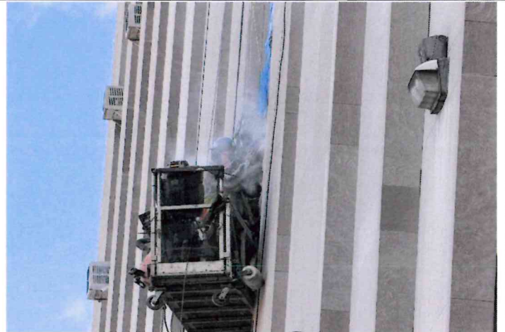
Photo 22: Courthouse 3rd Floor Infill grinding, 12/6/24
