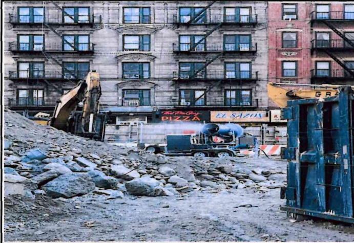
Photo 3: Crushed concrete Stockpile looking east, 11/13/24
