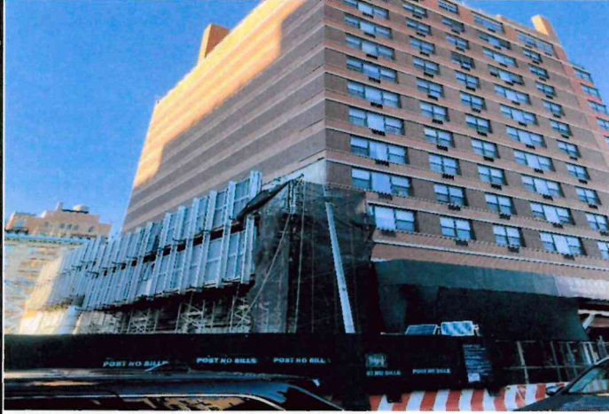
Photo 13: View of North Tower Gym Wall removal, 11/13/24
