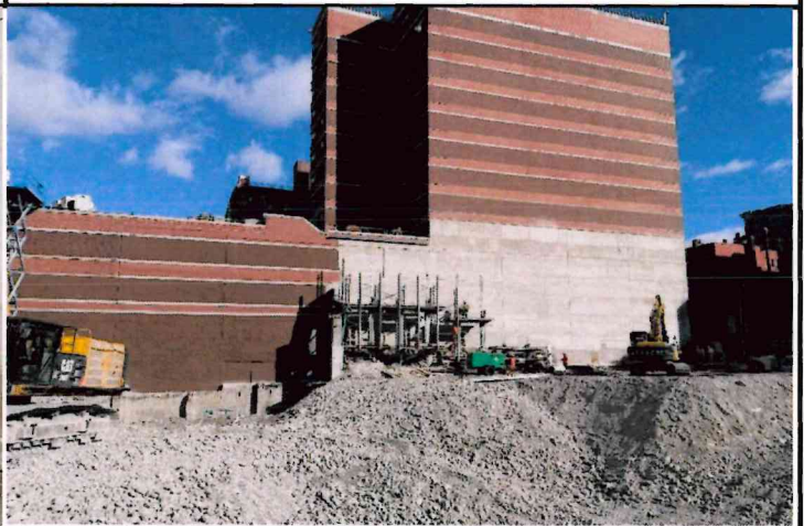
Photo 16: View of North Tower Gym Wall removal, 12/6/24
