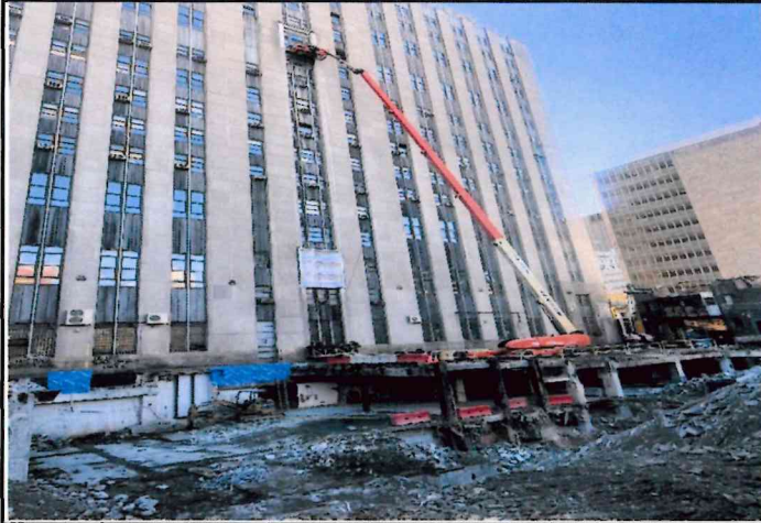
Photo 5: Courthouse Sally Port & 12th Floor Bridge Infill, 11/13/24
