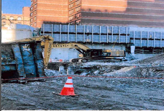
Photo 1: North Tower basement debris removal, 11/13/24
