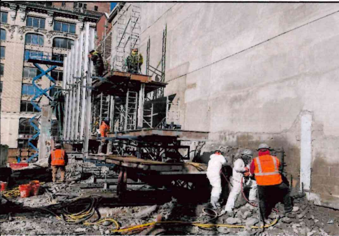
Photo 15: View of North Tower Gym wall removal, 12/6/24
