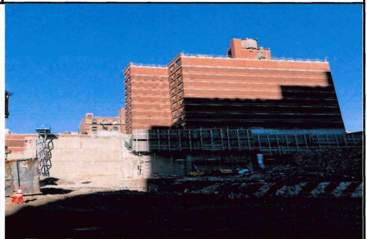
Photo 8: View of North Tower wall removal adjacent to Chung Pak, 11/13/24
