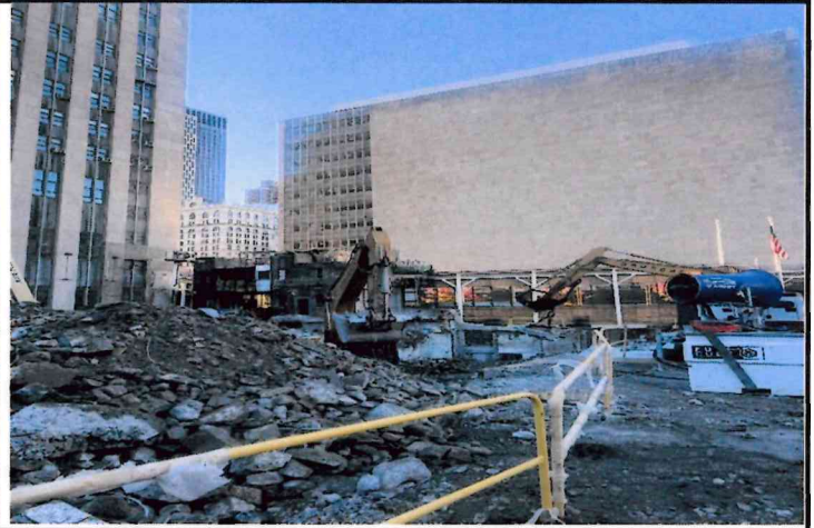
Photo 6: South Tower basement debris removal, 11/13/24
