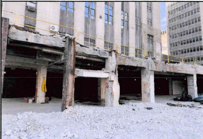
Photo 19: View of Sally Port adjacent to Courthouse, 12/6/24
