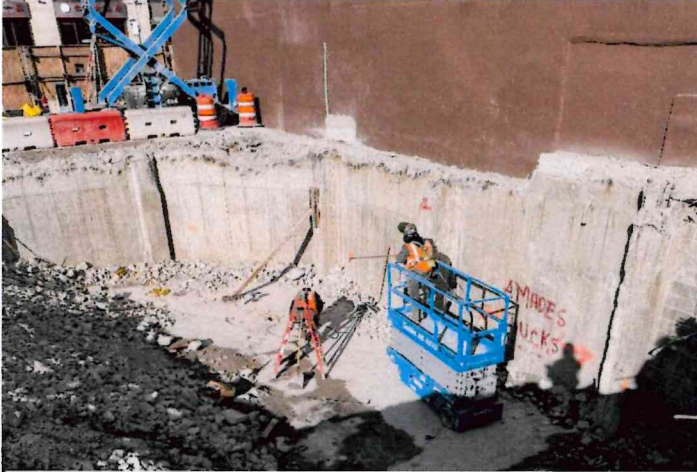
Photo 17: View of Chung Pak Bldg. Water Proofing, 12/6/24
