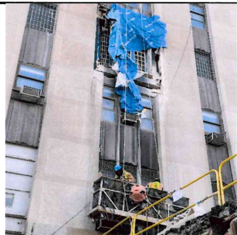
Photo 20: View of Courthouse 3rd Floor Infill, showing "blue skin", 12/6/24
