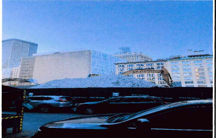
Photo 14: View from Baxter St. showing concrete pile, 11/13/24
