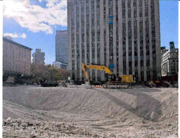
Photo 18: View of crushed concrete placement, 12/6/24
