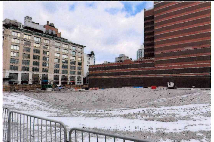
Photo 8: View of Chung Pak south wall showing North Tower Gym Wall removed and filled former basement area, 1-28-25.
