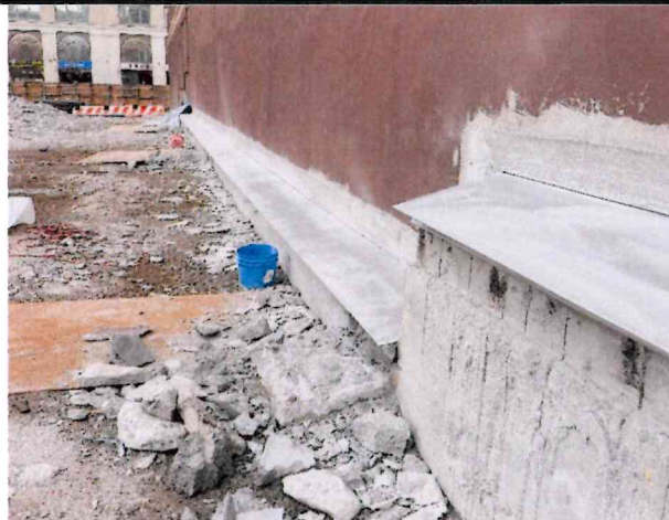
Photo 10: View of south wall Chung Pak building showing flashing installation, 1-28-25.
