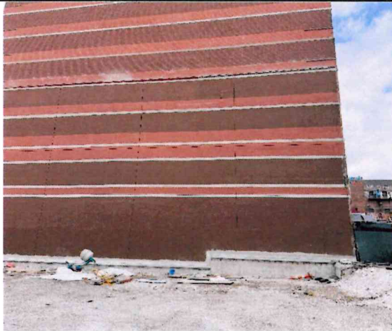
Photo 7: View of Chung Pak building south wall showing North Tower Gym Wall removed & flashing in progress, 1-28-25.
