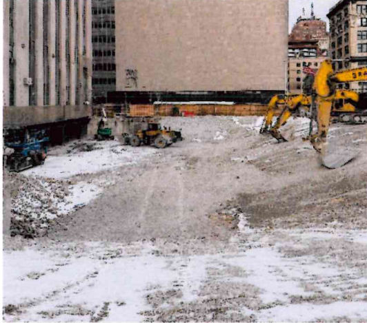
Photo 5: View of southeast corner of courthouse showing filled South Tower basement area, 1-28-25.
