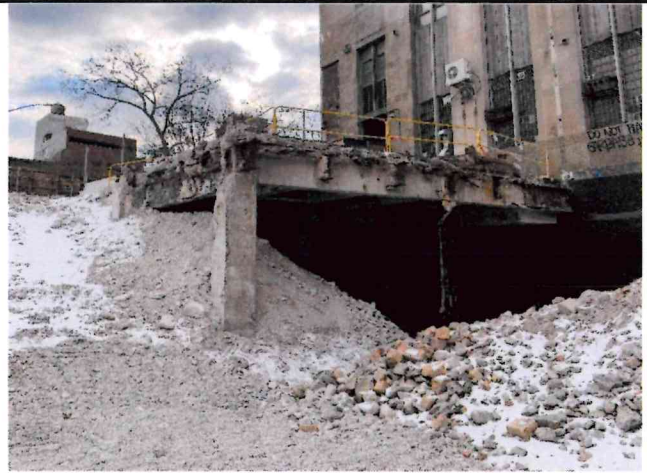
Photo 4: View of southeast corner of courthouse showing remaining concrete structure to be dismantled, 1-28-25.
