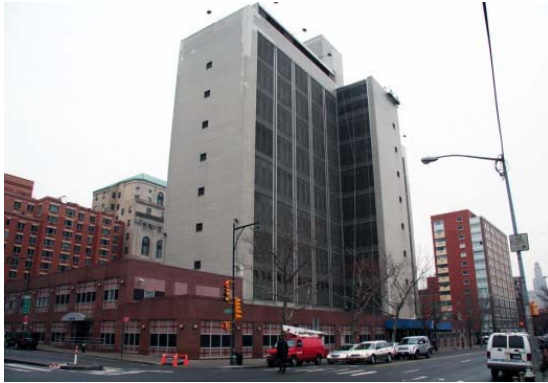
Brooklyn Detention Complex 275 Atlantic Avenue Downtown Brooklyn
